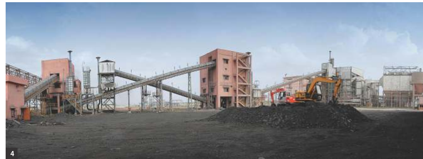
1. Power Plant Control Room 2. Tube Bending Machine 3. Floor Type Horizontal Boring Machine 4. Power Plant
